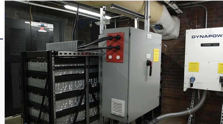
Statehouse backup battery (Green Mountain Power)
